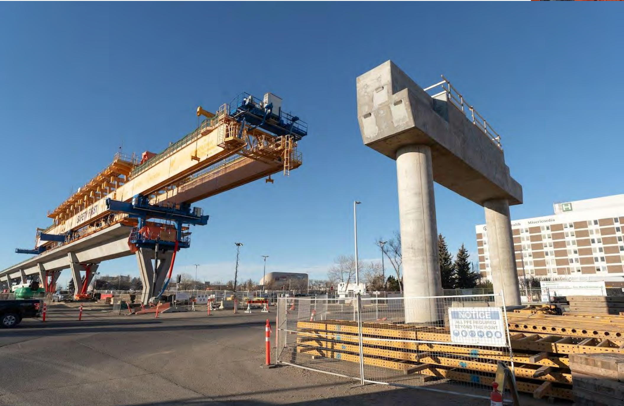
87 Avenue Elevated Guideway
